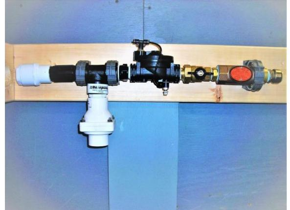
**STEP #2:** Install the Suction Pipe by using either 45 or 90 deg. elbows if necessary.
