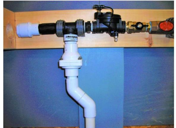
**STEP #3:** Install the Discharge Pipe using either rigid PVC pipe or the supplied hose or both.
